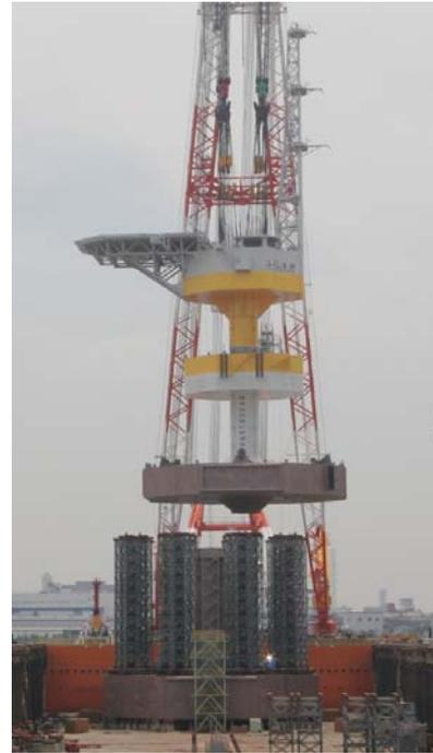
Fig. 12. Installation on lower hull
